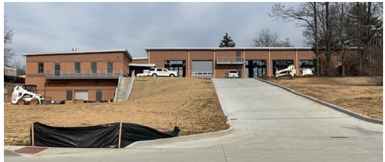
Rear of new firehouse facing Western Reserve Road
