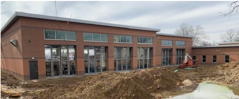
Front of new firehouse facing Overlook Drive
